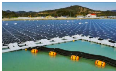
Figure 7. Floating photovoltaic (FPV) systems in Hyogo, Japan (Galdino and de Almeida Olivieri, 2017)
